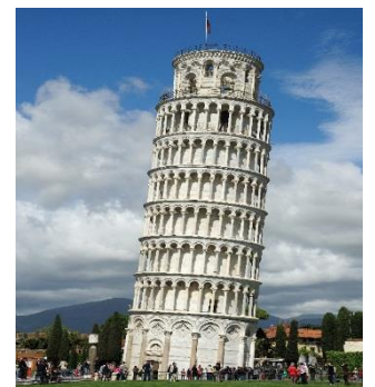
Leaning Tower of Pisa
